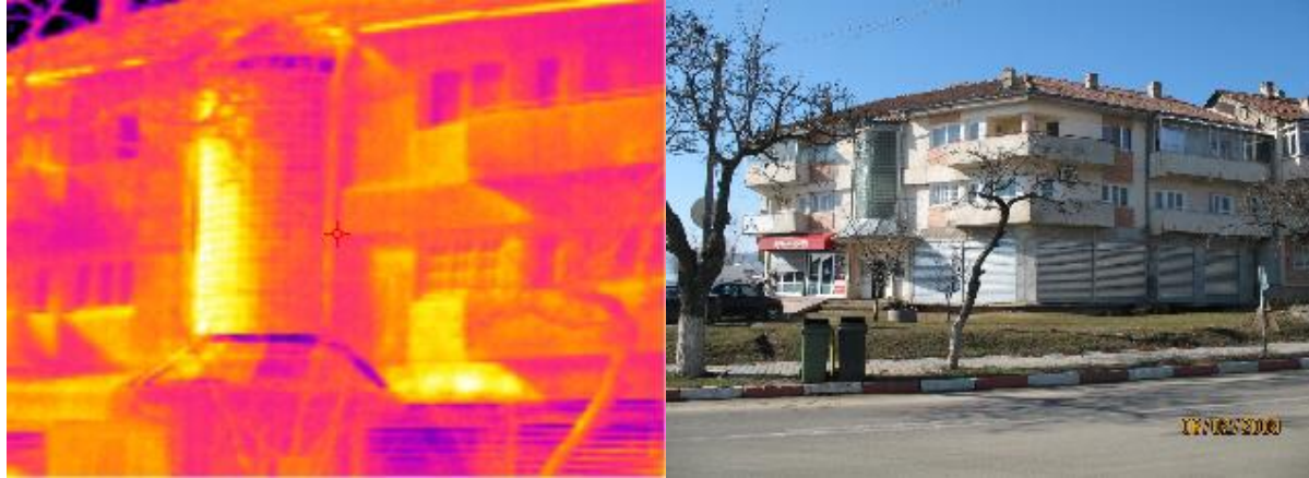
Thermal and visible image
