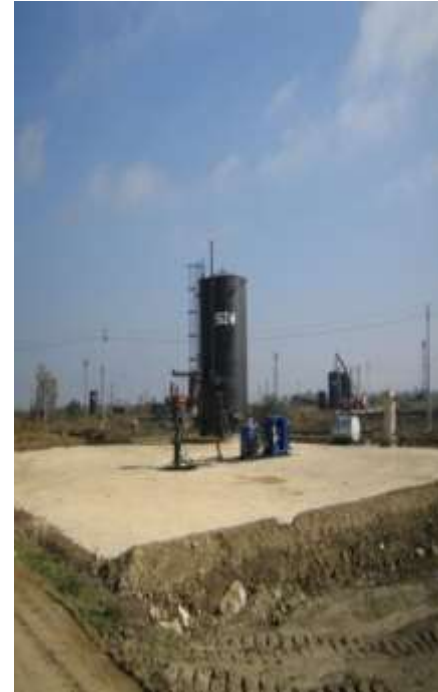
Bankers Re-activated Well Site
