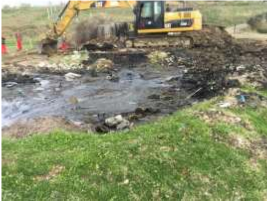
Well site reclamation and remediation activities
