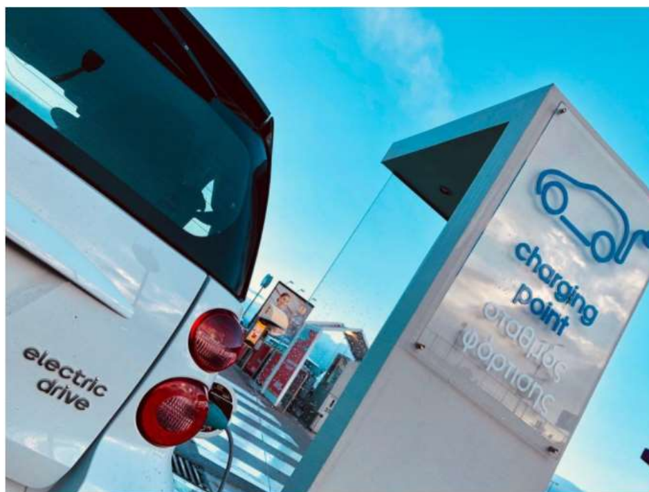
Figure 56 EV Charging Station in the parking area of Athens International Airport
